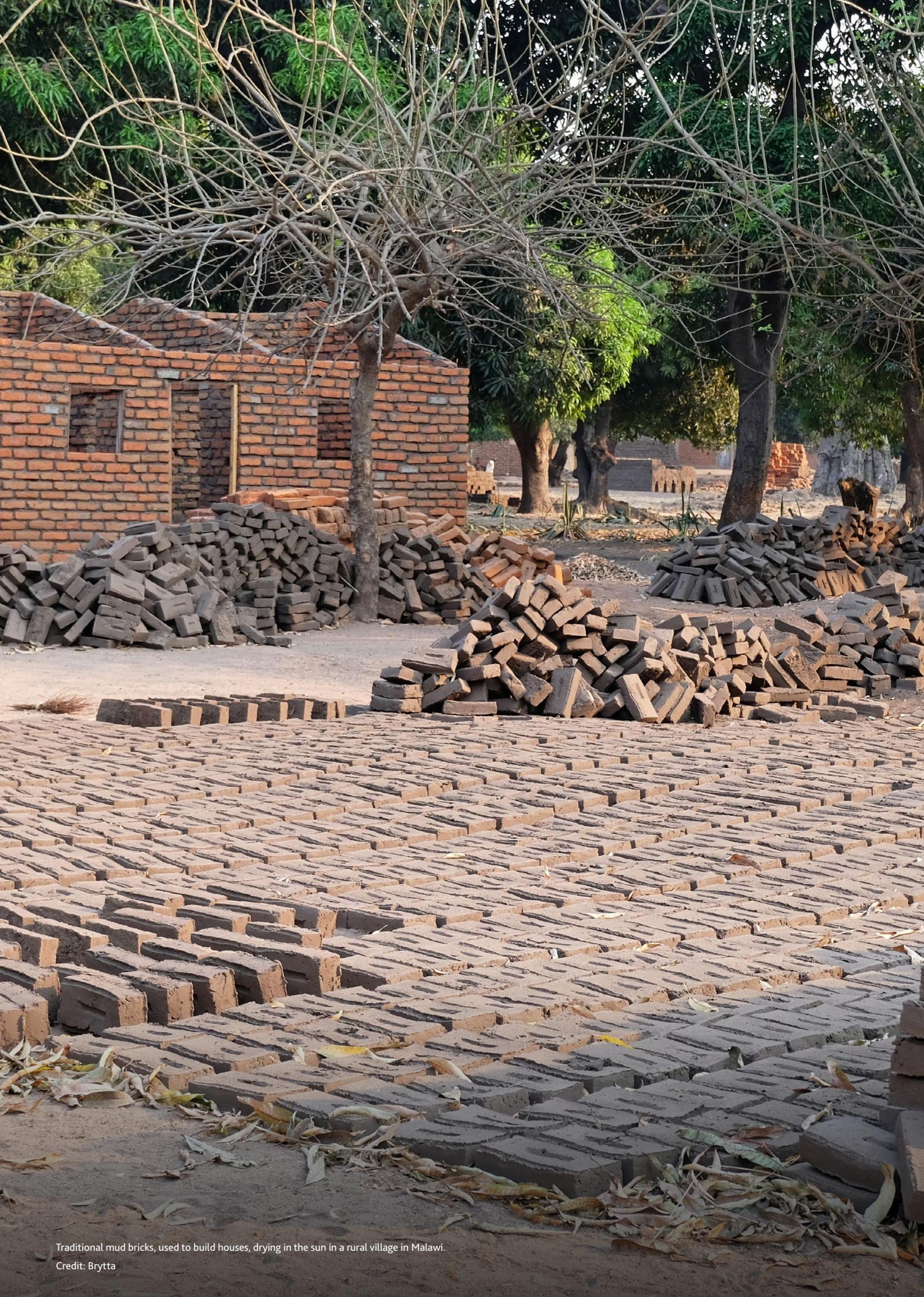
Traditional mud bricks, used to build houses, drying in the sun in a rural village in Malawi.
