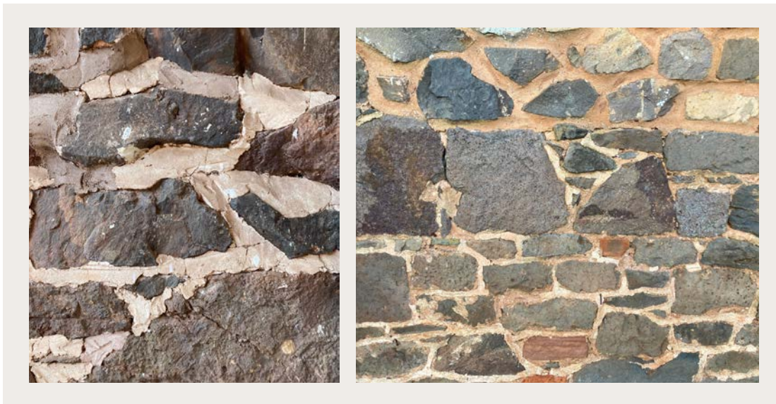
Figure 13: Photographs showing the use of cement mortar to repoint lime mortar at Killerton.
